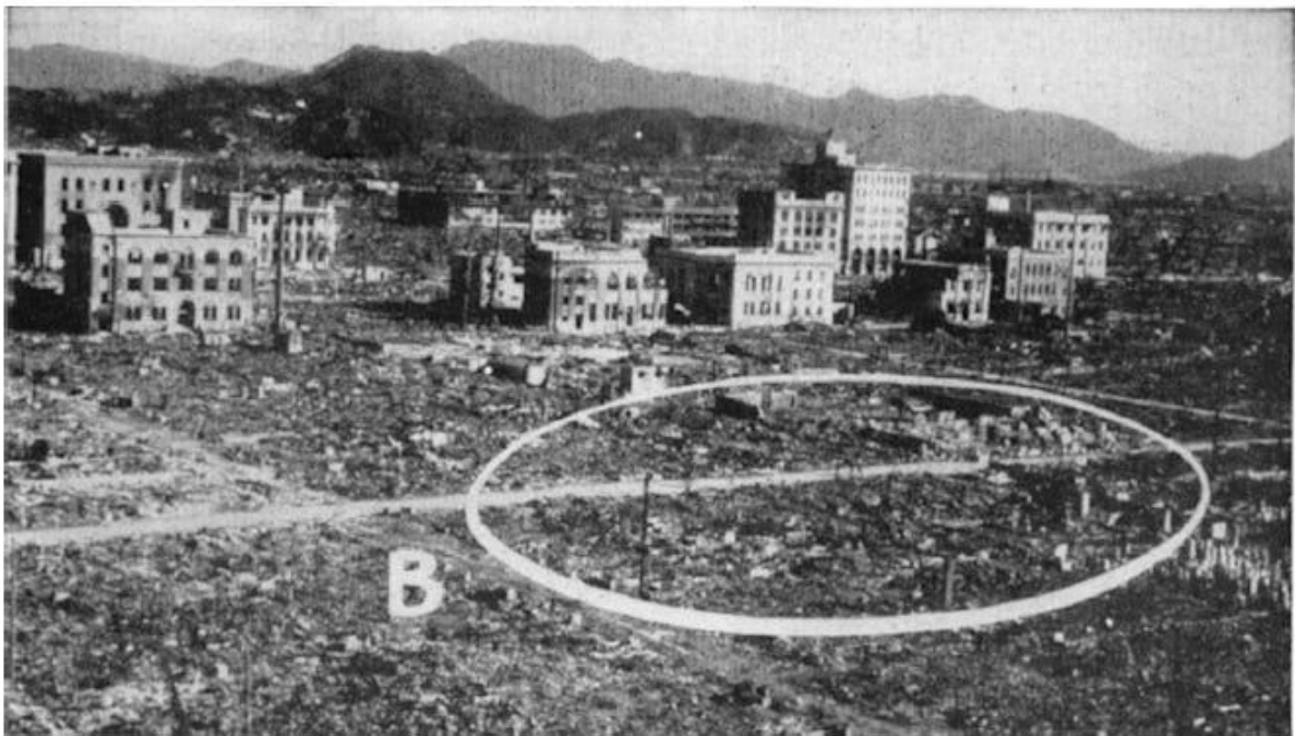
Figure 13.1 from Book: Photograph of downtown Hiroshima, taken by Alexander P. de Seversky during his visit in early September 1945. The original figure caption [5] reads as follows: “A cluster of concrete office buildings, standing erect and structurally intact amidst the ashes of the surrounding wooden houses, near ‘ground zero’ (B).”
