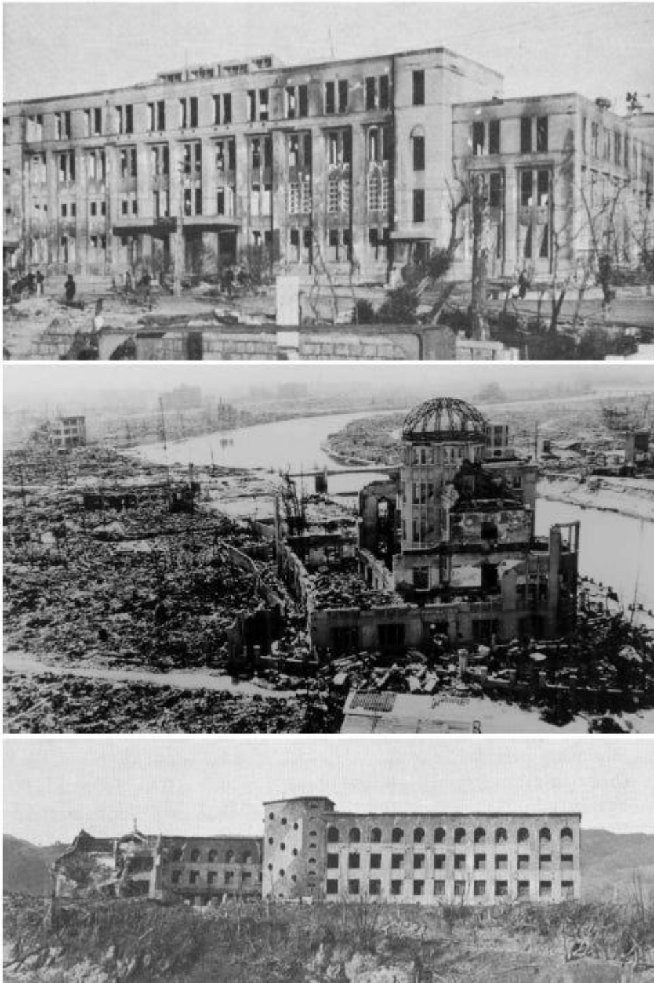
Figure 5.3 from Book: Three of many burnt-out buildings that according to various studies [82, 83] yielded pristine tiles or bricks suitable for measurement of gamma ray dosage by thermoluminescence. Top: Hiroshima City Hall; center: Hiroshima Prefectural Industrial Promotion Hall (now commonly called the 'Atomic Bomb Dome'); bottom: Shiroyama elementary school in Nagasaki.
